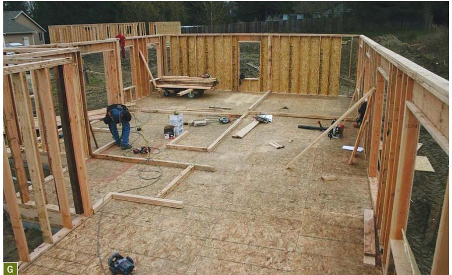
bobs have sped up this process considerably. I personally like to sheath the first-floor walls before heading up to the next level. This stabilizes the wall for the second floor deck assembly. With all of this accomplished, we've made room for the third delivery.
