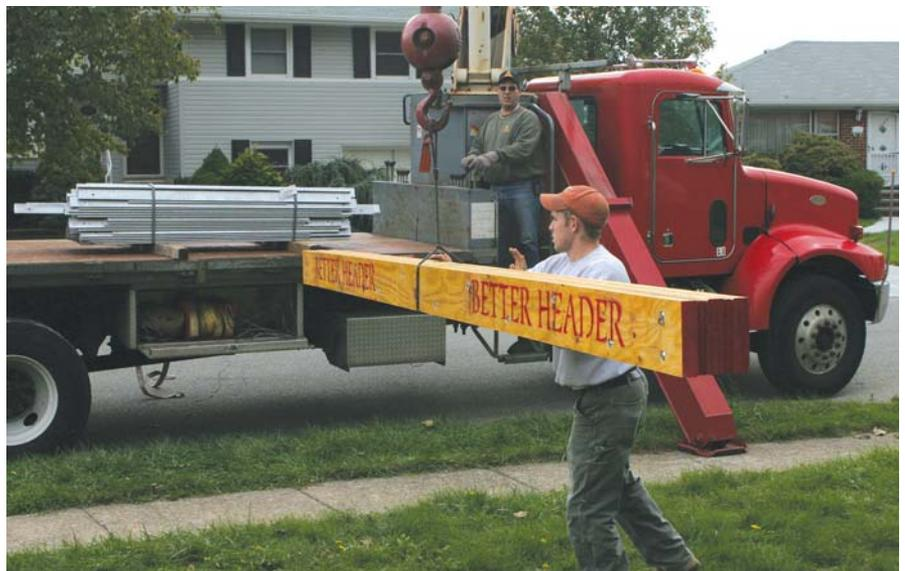
Setting the steel first, before any other deliveries, allows easy access to the work area.
