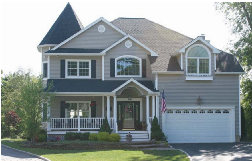
A construction calculator can help suppliers and builders alike navigate the maze of roof lines and pitches.
