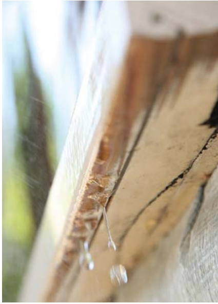
Create enough pitch on a sill, and a wide enough drip kerf, and water will not travel back under a sill or drip behind the siding.
